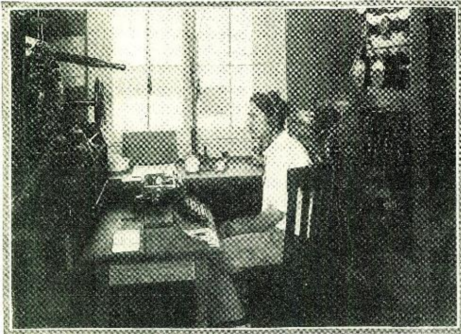
One of the “old stand-by” stations fully equipped with navy apparatus. The receiver is the faithful S.E. 143 with a DeForest vacuum tube control panel of early design. The transmitter is similar to the ones a number of boys are playing with now (self cleaning quenched gap an’ everythin!!) except it is a 5-KW affair.
