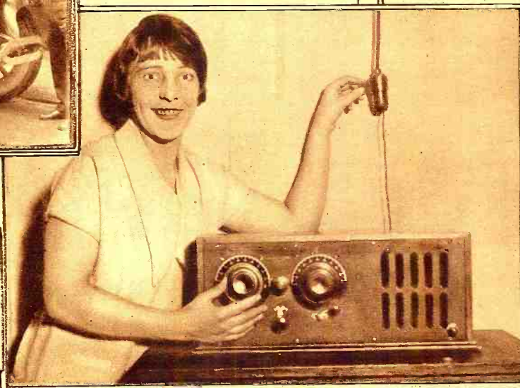
Right: Something new in radio sets. Gertrude Dalton and her unique broadcast receiver which requires no aerial, no ground and no "A" or "B" batteries. It works directly from the light socket. The loud speaker is contained in the right hand section of the cabinet. It is a three tube set and measures only 7 by 18 inches. © Fotograms, N. Y.
