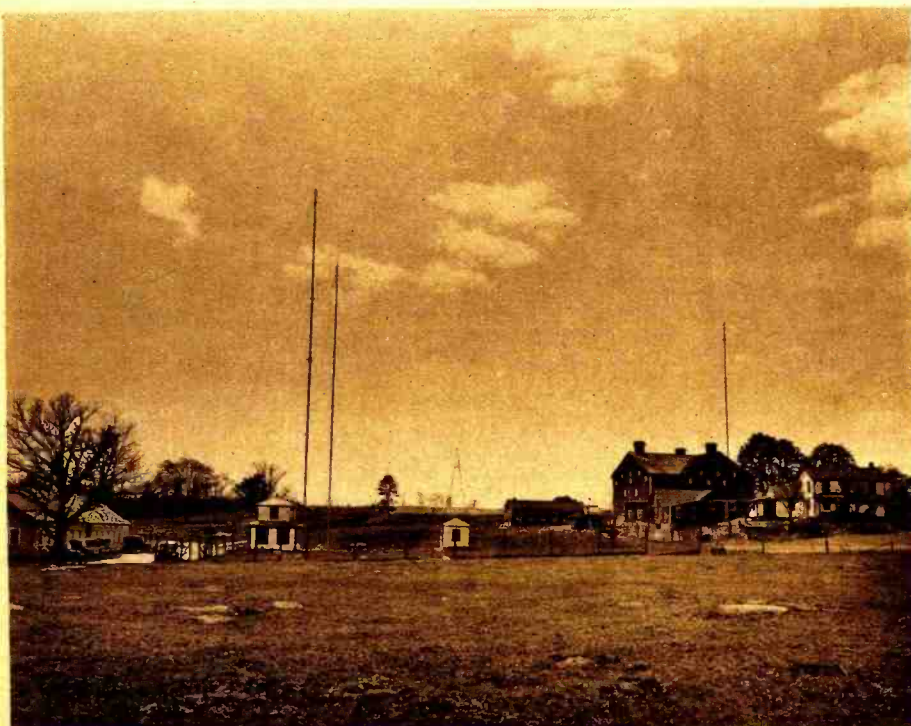
The radio shack and the two immense 100-foot towers which support the aerial of station 8BRC. Another aerial atop Mr. Myers' house is employed for broadcast reception.
