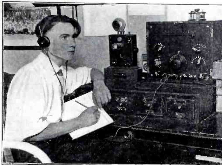
This Young Enthusiast Confines His Attention to Radio Telephony. He Has Secured Good Results Using One Vacuum Tube With a Plate Voltage of Only 40 Volts.
