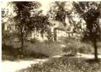
One of the many buildings
