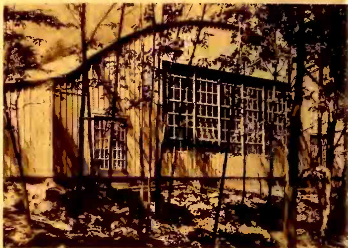
Also built by listeners' gifts is this pavilion, nearly completed, which will be used as a rest-house for the parties of pilgrims who frequently come to Graymoor.
