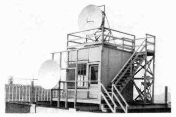
Figure 104. Permanent installation of microwave relay antenna.
