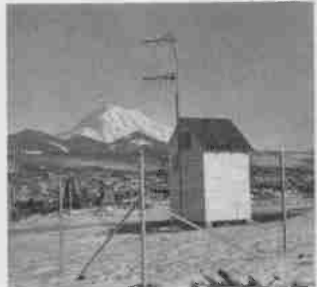
Typical repeater station located on a mountain for receiving signals from several radio-active snow gage stations and sending them on to the recording station.
