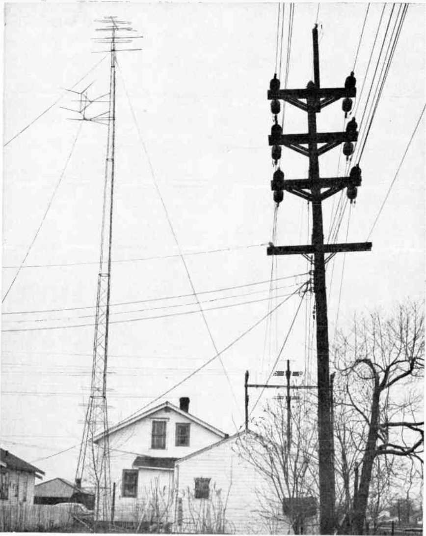
The installer and the owner of this installation are asking for trouble. If the mast should give way, it could fall onto high-tension lines in any one of three directions, and could set the house on fire or electrocute the occupants.
