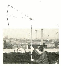
Wooden masts, made from broomsticks, made perfectly good suports for the simpler types of antennas in many cases. Shortages of steel masts have made these installation feasible in many TV localities.
