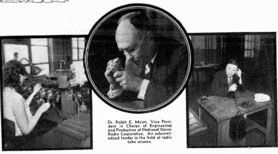
An operator working at one of the new National Union high speed stem making machines. She was formerly with Westinghouse Lamp Works and has had seven years experience in tube manufacture.
