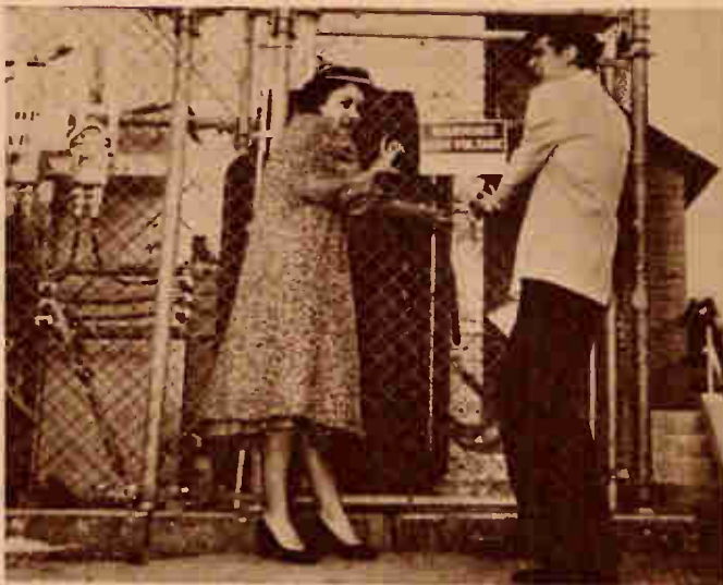
"'NO ADMISSION TO THE PUBLIC' signs were everywhere. A kindly engineer explained that much high voltage, dangerous equipment make ban necessary."
