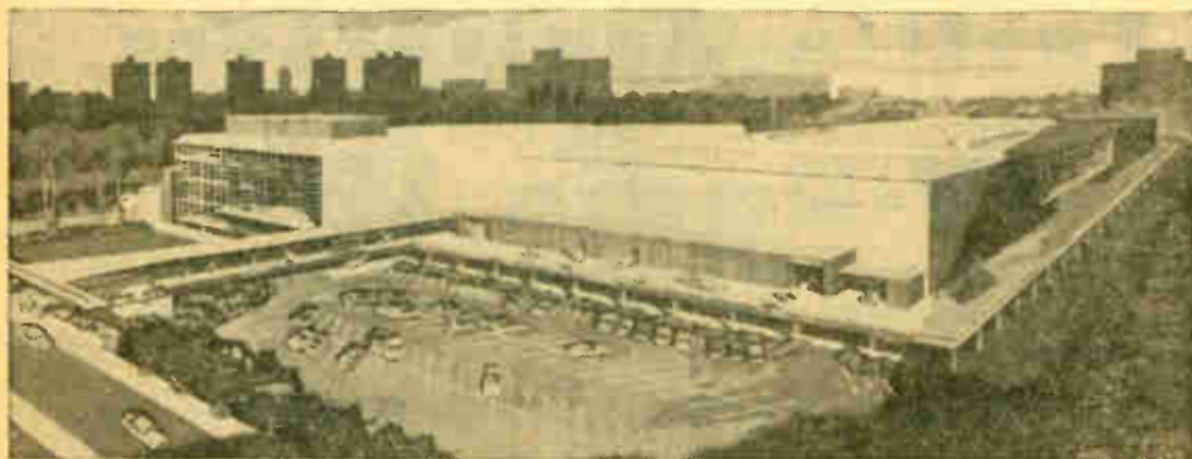
CBS TELEVISION CITY , the first plant designed exclusively for television, will look like this next October, when it is scheduled to begin broadcasting operations. Covering fifteen Los Angeles acres, this initial unit will house four mammoth studios and three rehearsal halls in the section at right, with the glass-fronted four-story unit at left serving as the administration building. The ramp running around the second story of the studio area will be used to haul scenery, which will be designed and constructed in shops in the far end of the administration building. When finally completed, the project will cover thirty-five acres.
