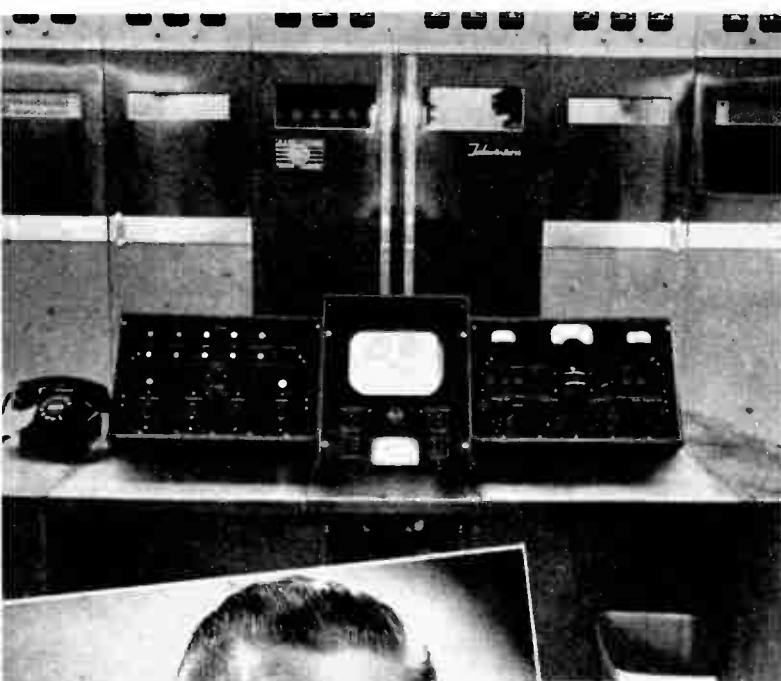
▲ AN ACTUAL PHOTO of the test pattern on the master control monitor at the KNBH transmitter on Mt. Wilson. KNBH's Channel 4 is at a frequency of 66-72 megacycles, with a video power of 27.5 kilowatts, and audio power of 13.75 kilowatts. (NBC-Zeigler photo.)
