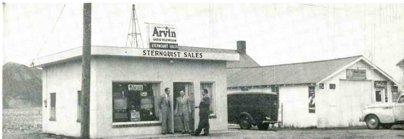
• Sternquist erected this tidy radio-TV sales room alongside the auto service shop he started 20 years ago.
