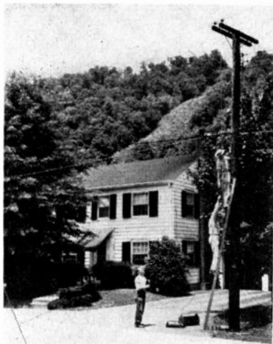
• Tapping into the main cable line was a simple matter.
