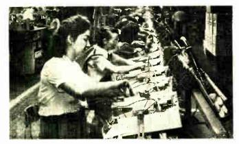
Wiring and soldering of component parts on the production line before conveyor belt takes chassis for early test.
