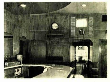
Note multiple viewing units in this television orrangement. Screen above the door is designed to fit in with woodwork. Second viewer is in side room beyond. Remote control unit is behind the bar to left.
