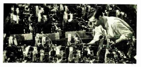
Television chassis are intricate pieces of mechanism. Receivers have from five to six times more tubes than the ordinary radio set. An inspector like the one above must test each chassis before passing it along to cabinet assembly.
