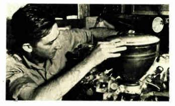
During brief sojourn chassis gets finishing touch with insertion of 10-inch cathode-ray tube and alignment of IF-RF.
