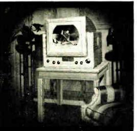
THE AMBASSADOR— Table model with 16" metal direct-view tube. 31 tubes plus 2 rectifiers. AM-FM radio.
