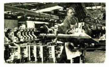
Chossis is unloaded from belt and rests for inspection at end of one leg of journey. Cabinet assembly follows.
