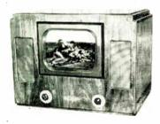
This receiver features a 12-inch picture tube and a device called the "Mars Dual-Tuner", which is said to eliminate consumer confusion in tuning. Ordinarily the consumer is faced with several dials, but this set has only two dials; one for station selection and the other for sound and picture control. The picture tube is independently mounted and never has to be removed in case of servicing.
