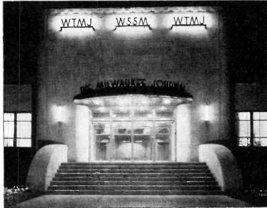
MILWAUKEE'S new Radio City, where W55M makes its home. A 50,000-watt transmitter, located on hilltop outside of the city, supplies noise-free reception for listeners within seventy-mile radius. The FM studios at the WTMJ-W55M Radio City are the last word in acoustical efficiency
