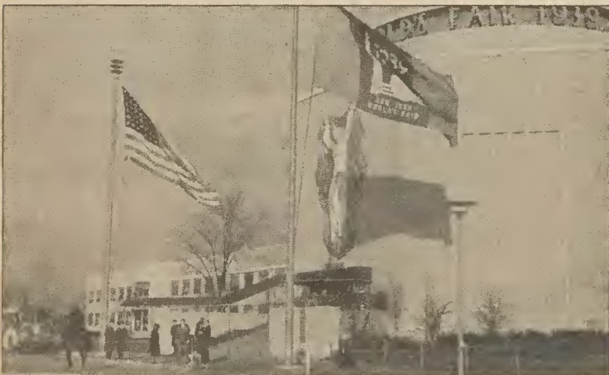
The Fair's Administration Building is the center of world-encircling exposition activities, houses 700 specialized workers. Sculpture above entrance portrays Mithra lifting veil which obscures the "World of Tomorrow"
