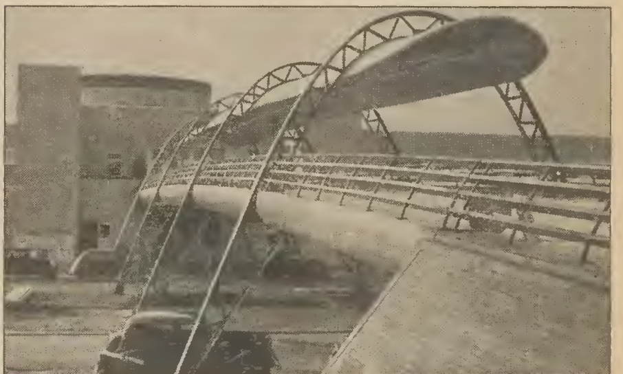
Yacht-like in its lines is this "Bridge of Tomorrow," connecting the Administration Building with exhibit zones. Its "hull," rails and abutment are of clear, varnished fir; steelwork is painted "New York City Blue"
