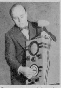
The resonoscope tests pitch, can also be used with great accuracy for tuning all kinds of musical instruments
