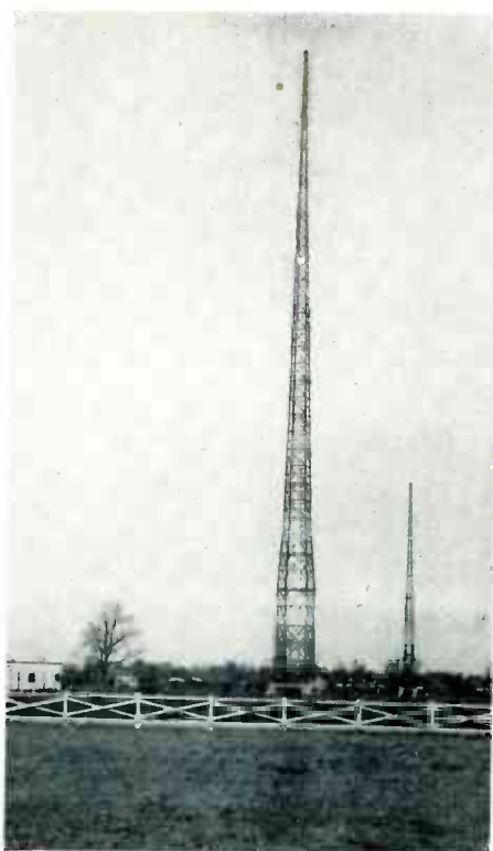
Fig. 10. Six-Layer FM Antenna at WBRL, Baton Rouge, on AM Tower.
