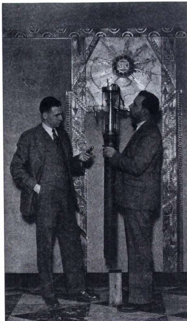
100-kw tube compared with small receiving type.
