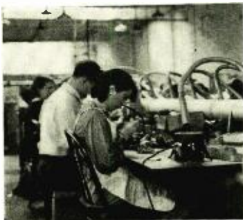
Removal of fumes from solder and glue pots.
