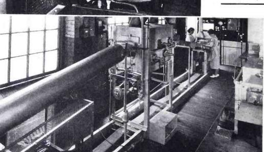
WELDING EXHAUST TUBULATION TO HEADER. A POWERFUL THYRATRON-CONTROLLED WELDER FUSES THE OPEN LENGTH OF METAL TUBING TO THE HEADER.
