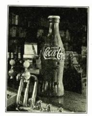
stands two feet high, is molded in two pieces of General Plastics' Durez, brilliant scarlet in color, and is equipped with Crosley's standard 165 chassis, using five tubes. The lettering of the words "Coca-Cola" forms the grille over the dynamic speaker. and the translucent green dial is lighted from behind. Tone value and volume are reported good.
