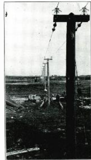
Fig. 5. View of transmission line from transmitter end.
