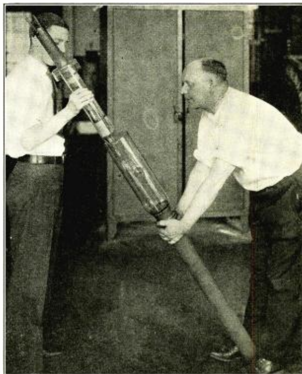
Fig. 3. Assembling a type 862 tube.
