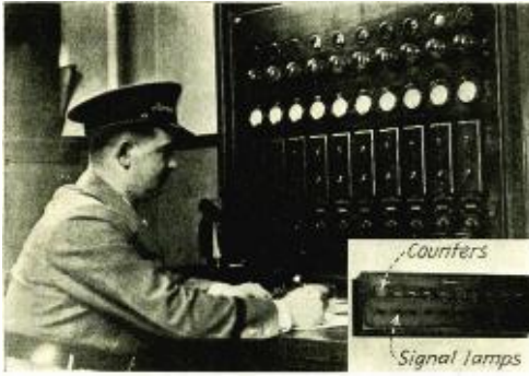
Bakelite laminated control board of the "electric eye" in the supervisor's office. Lower right—Indicator panel of phenol resinoid. The frequency with which the light goes on and off shows the traffic density of a particular lane
