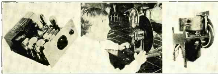
Fig. 5. Radio receiver. Fig. 6. The radiovisor. Fig. 7. Scanning drum and mechanical shutter radiovisor.
