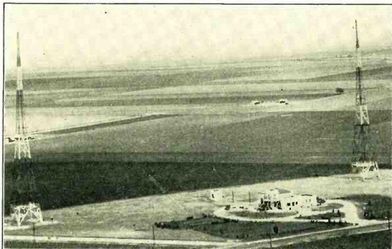
Fig. 15. General view of WFAA, Dallas, Texas.
