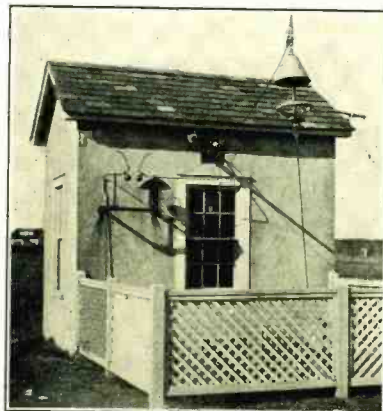
Fig. 14. Tuning house, antenna down lead and lead-in, WEA F.
