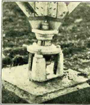
Fig. 13. Close-up view of insulated tower footing.
