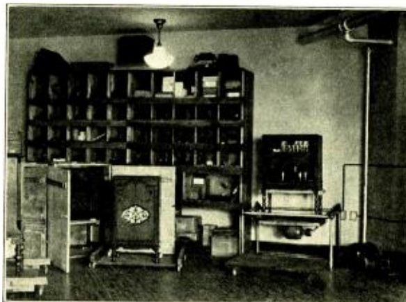
Fig. 5. Stock bins. To the right, the vibrator.
