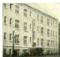
A Doctor's Call System in the Virgin-Pearl apartments, Buffalo, New York, provides service to the private offices through two Powerizer 250 and one Powerizer 171 amplifiers, plus sixteen magnetic speakers. Installation by Buffalo Radio Engineering Laboratories.
