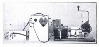
View of the combination receiver-oscillator and mechanically driven tape recorder employed for obtaining altitude readings. The records indicate the altitude of the plane from the surface of the earth rather than the sea level.
