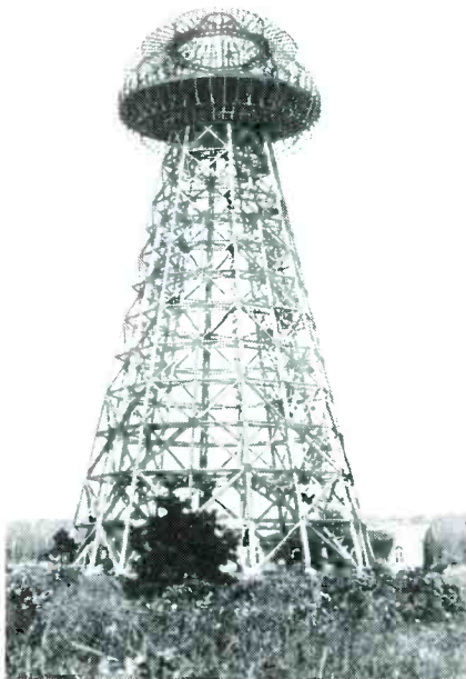
Located in Shoreham, NY, this tower was built by Tesla for experiments in world-wide telegraphy and power transmission. The tower never became operational.
