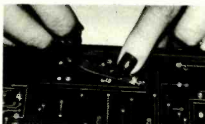
FIG. 9—USING SELF-ADHESIVE copper foil to make a repair.
