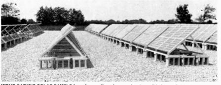
WBNO RADIO'S SOLAR PANELS face due south and cover about one-third acre. Cables leading from each panel connect to the computer-control center where the power is distributed, first to the AM transmitter, then to storage batteries. Any surplus power is used for station lighting, teletype machines, the AM console, etc.
