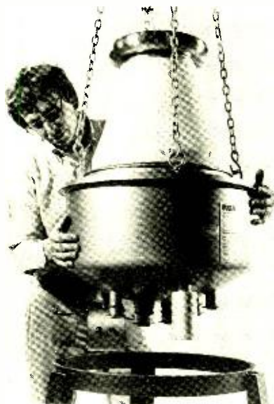
320-POUND VACUUM TUBE designed by RCA switches 25 MW—enough power to turn on 300,000 TV sets—and will be used in Princeton University nuclear fusion tests. Computers were used in designing the tube, constructed by engineers of RCA's department of Electro-Optics and Devices in Lancaster, PA.
