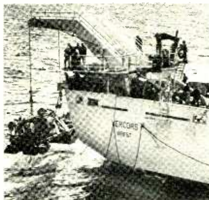
UNDERWATER SEA PLOW is suspended from the stern of the French cable ship Vercors , that has plowed under—in a trench about two feet deep—the parts of the transatlantic cable that lie in shallow water on the continental shelves off the U.S.A. and France.
