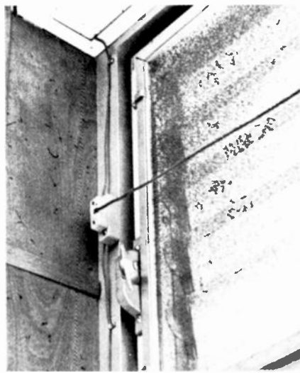
LAUNDROMAT INSTALLATION INCLUDES SOME HARD-WIRE PROTECTION. Trap-type switch on over-door transom is "supervised" — tamper-resistant method of wiring that triggers alarm if circuit is bridged or opened, either one. Circuit from foil on door, and from smoke and heat detectors (not shown) operate out of same central control box. Sets off loud electronic sirens. Could be hooked to automatic telephone dialer to call owner, alarm company, police or fire department, or security guard.
