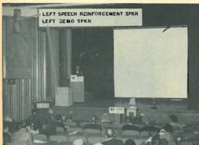
The hall as viewed from the console operator's position. Two more speakers are used on right of stage to balance system.
