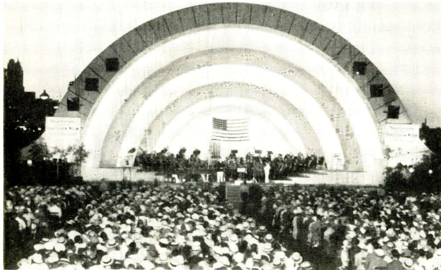
Photo A—Open air orchestra with inverted acoustical bowl which projects sounds over a large audience without electronic amplification.
