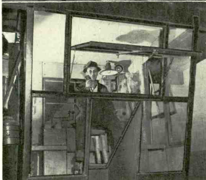
Carrier (wired) radio system used on moving overhead cranes lets operators handling material within the plant talk to other operators and personnel at ground stations to coordinate all crane operations.
