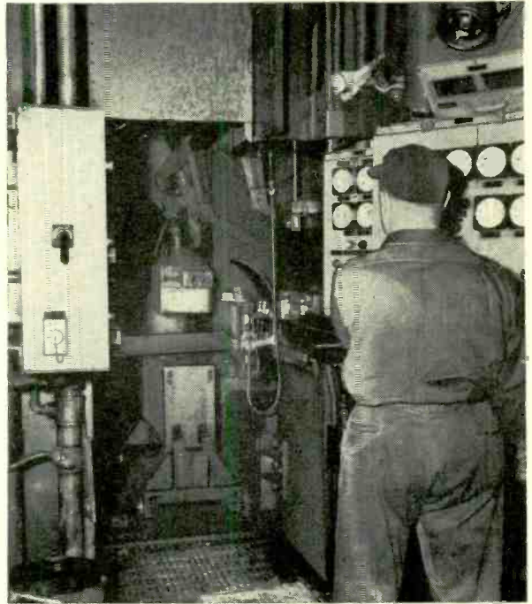
X-ray machine at the No. 7 tandem mill controls the rolling operation of the 54-inch strip-steel department. The device automatically keeps the gauge of the steel being rolled within the desired tolerance.
