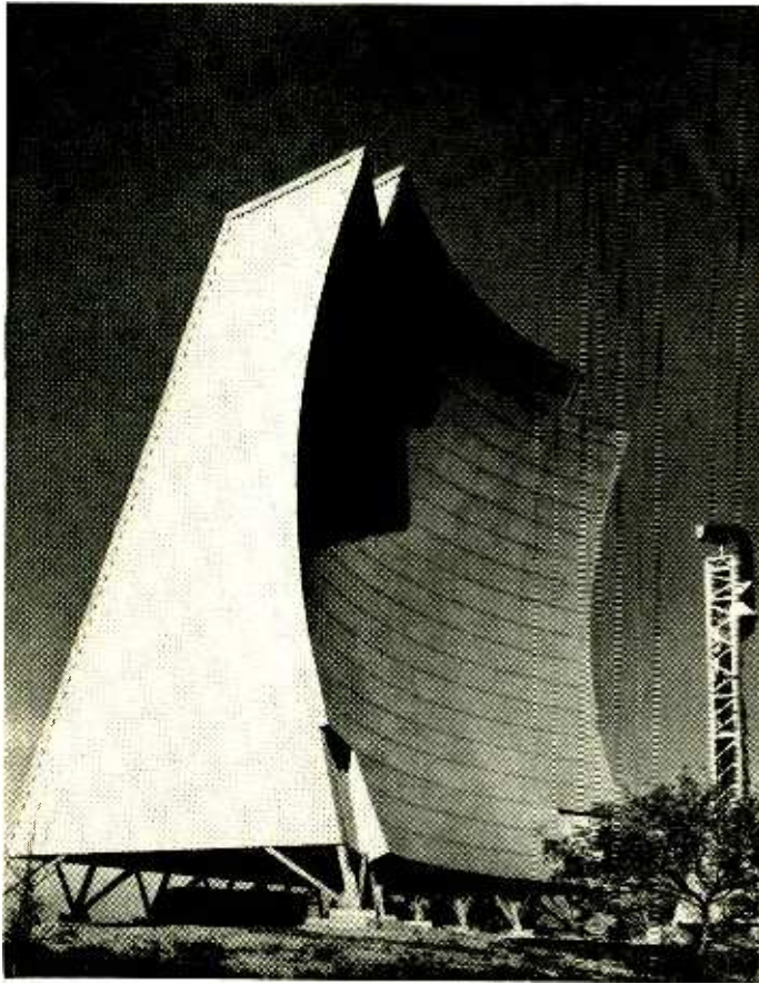
Giant over-the-horizon antenna designed by Bell Telephone Laboratories for "White Alice," Air Force Alaskan defense communications network.
