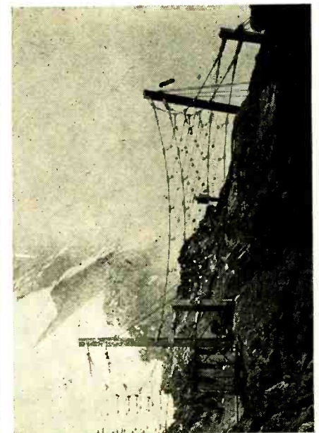
A close-up of the antenna system seen in the photograph at the top of the page. Antennas are supported on yards extending from the mountain, and held by guys to the rock above. (Antennas extend downward, but the guys go up!)
