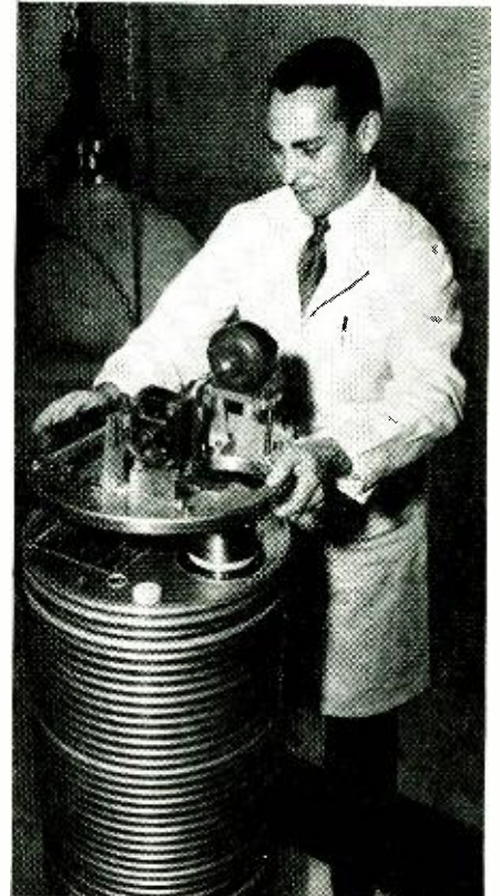
Putting the top assembly in place. Pressure tank can be seen in background.
