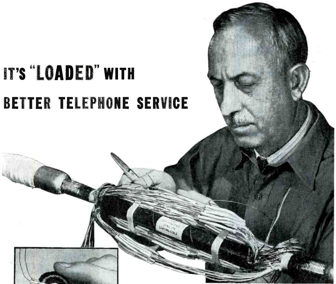
Twenty of the Bell System's newest small loading coils—like the one at the left—are housed in the long black case, mounted in a cable splice. This type of installation permits the economical extension of city cables to serve out-of-town subscribers.
