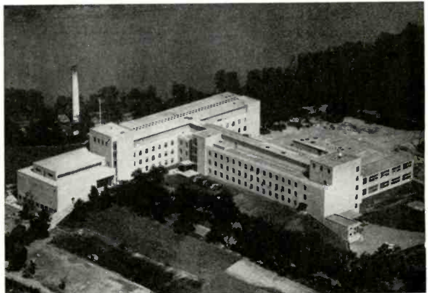
An overall view of G-E's new research laboratory building at Schenectady N. Y.
