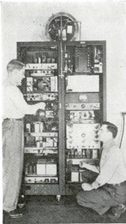
A rear view of the atomic time control unit.
