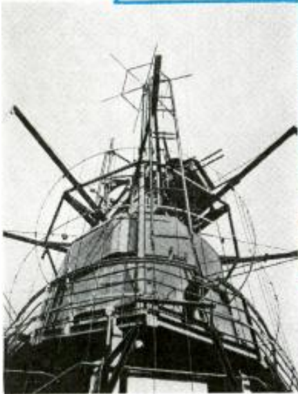
The Eiffel Tower bristles with TV antennas. Ladder enables workmen to reach the elements.
