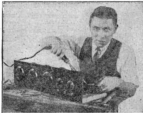
Front View KD-50, Neutrodyne Being Assembled
