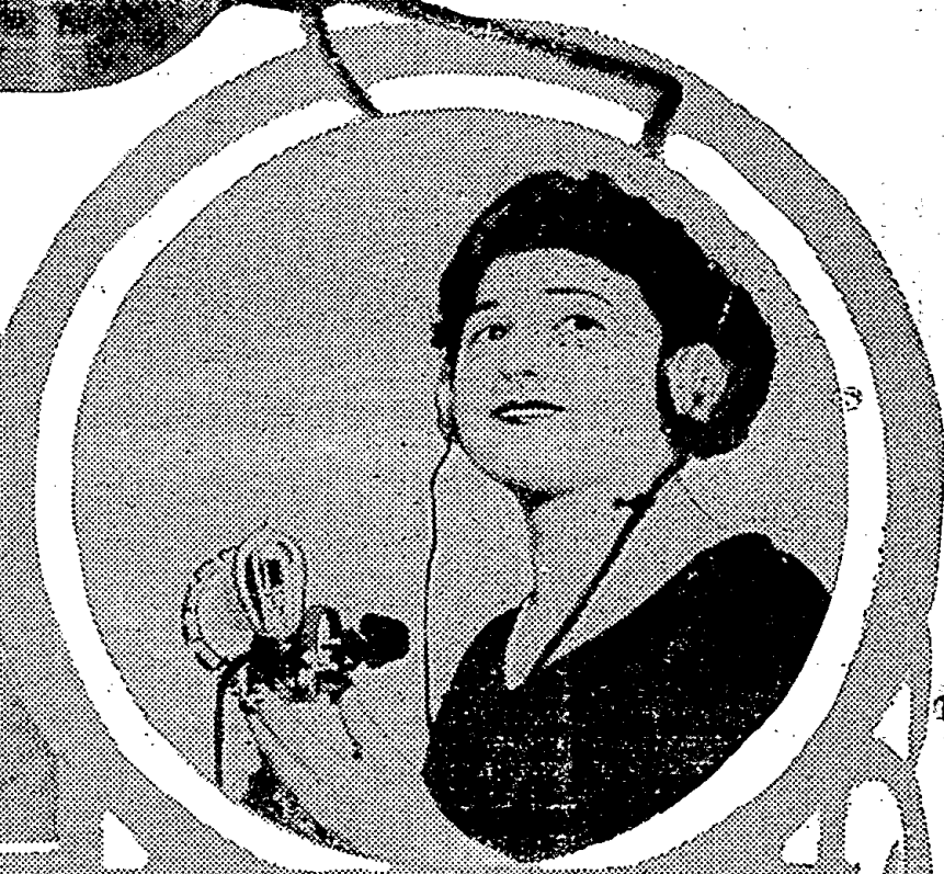
The amateur receiving set contest now in progress at the Radio Fair at the Hotel Imperial, New York City, has drawn entries from all parts of the country among which are many unusuals. Above is a novel entry in a vacuum tube set with spider web inductances, all mounted on the base of a standard audion socket © Newsreel
