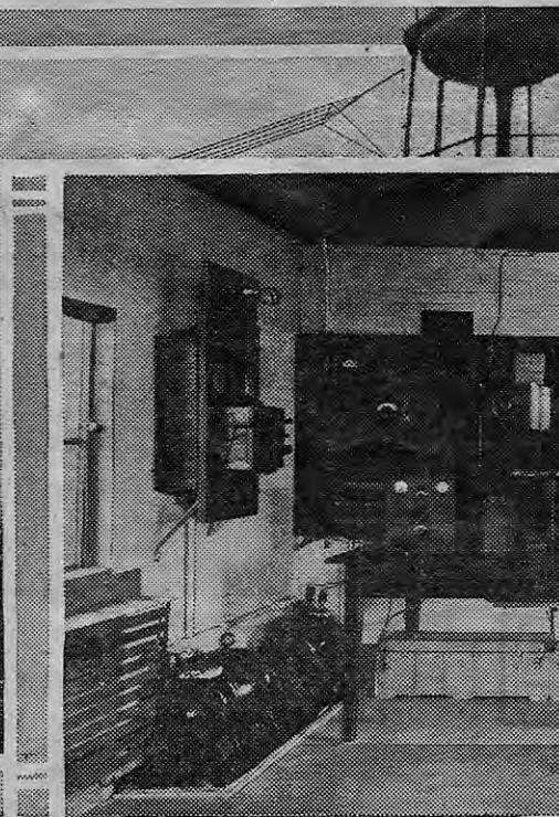
Cabin, antenna and mast of WWI, Dearborn, Michigan. The high end of antenna is supported by water tank. Below shows equipment.
